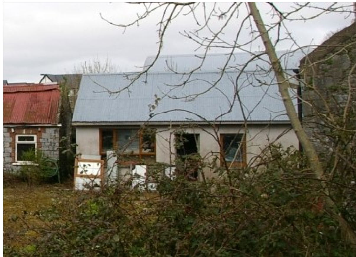
Plate 25: Southern elevation of modern structure Building D
