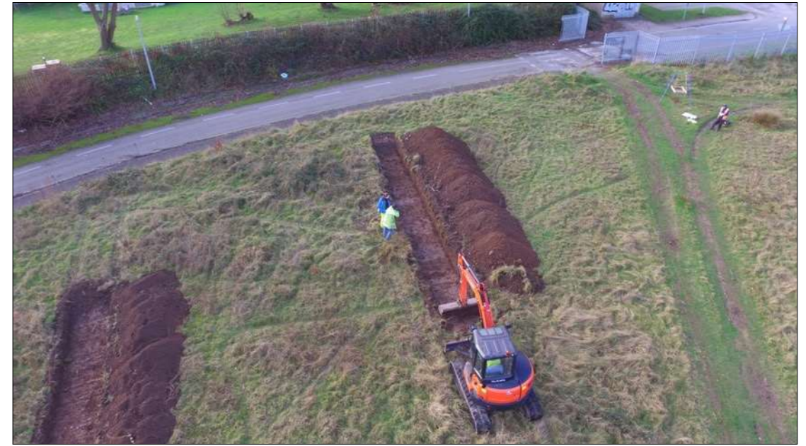
Plate 11 Trench 4, mid-ex, looking northwest
