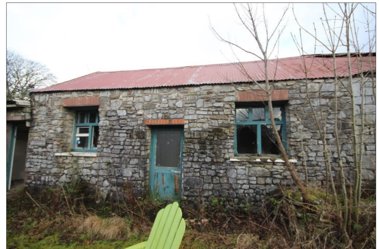
Plate 31: Southern elevation of Building F
