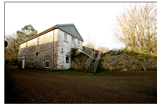
South-eastern and south-western elevations of Building A
