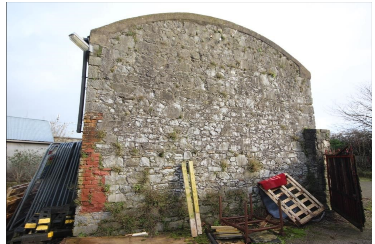
Plate 15: Southern elevation of Building B
