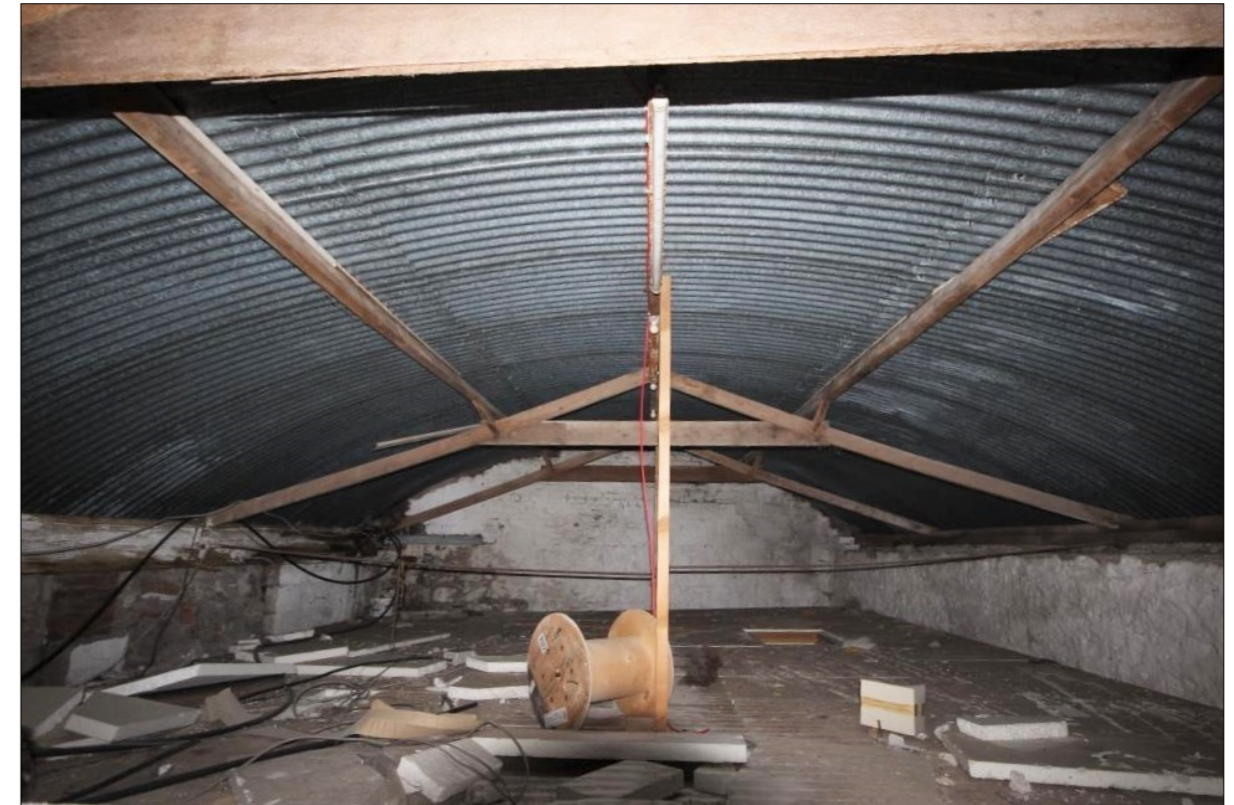
Plate 22: First floor room B-GF Building B
