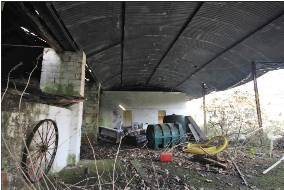
Plate 40: Interior of eastern portion of Building H looking north with modern concrete addition
