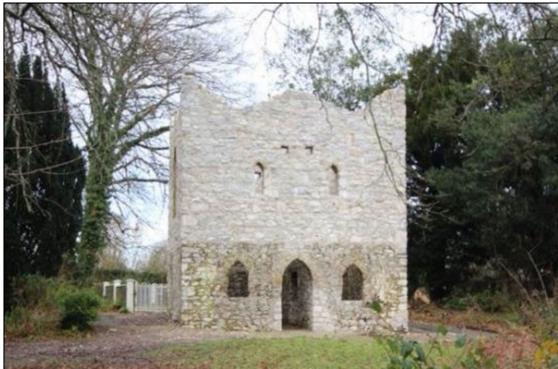
Plate 10.26: View from south of Folly in southeast end of Bessboro property following partial demolition and rebuilding (outside subject lands)
