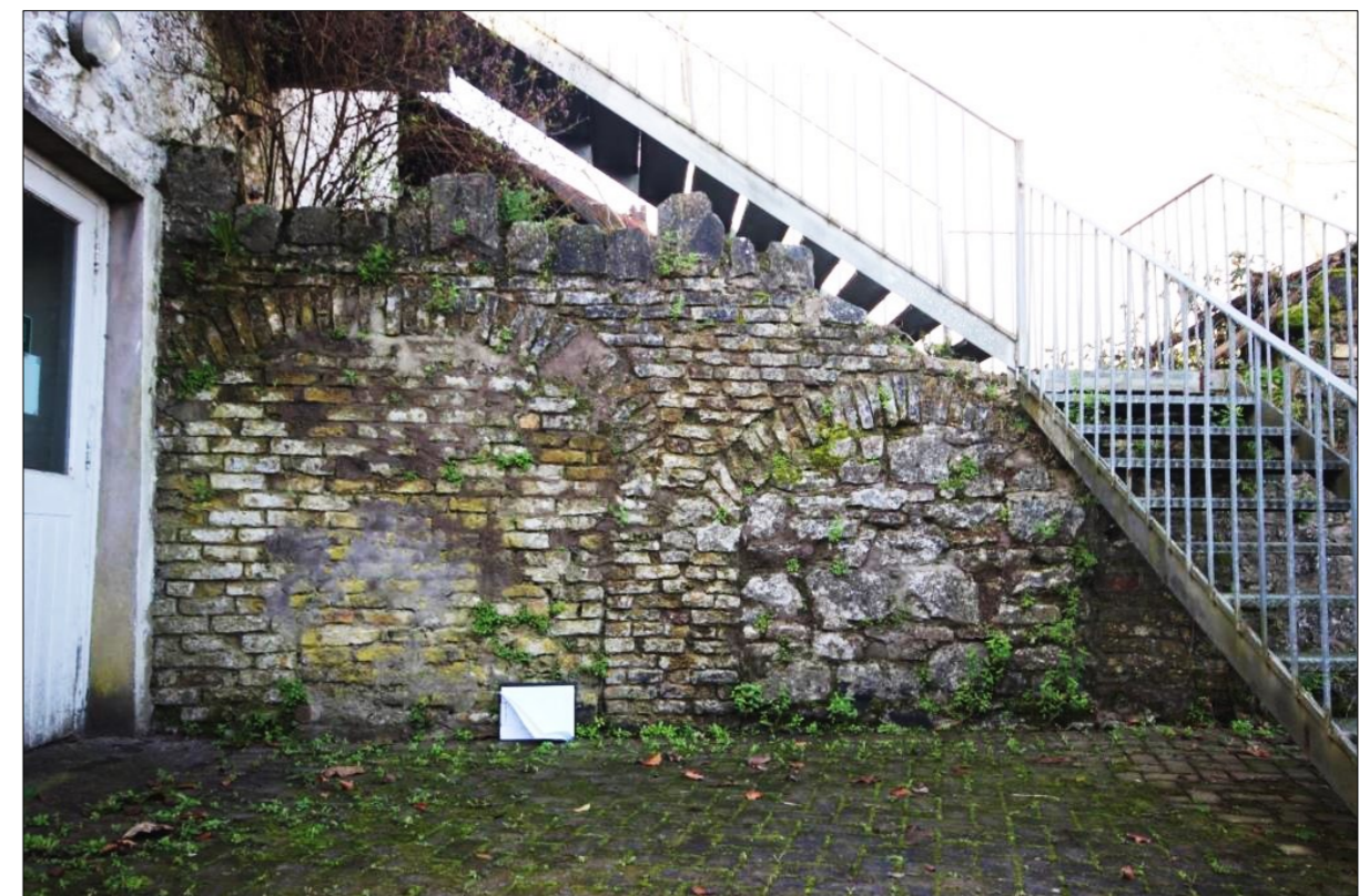
Plate 7: Blocked up brick arches in boundary wall to east of Building A
