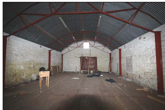
Interior looking north-east
