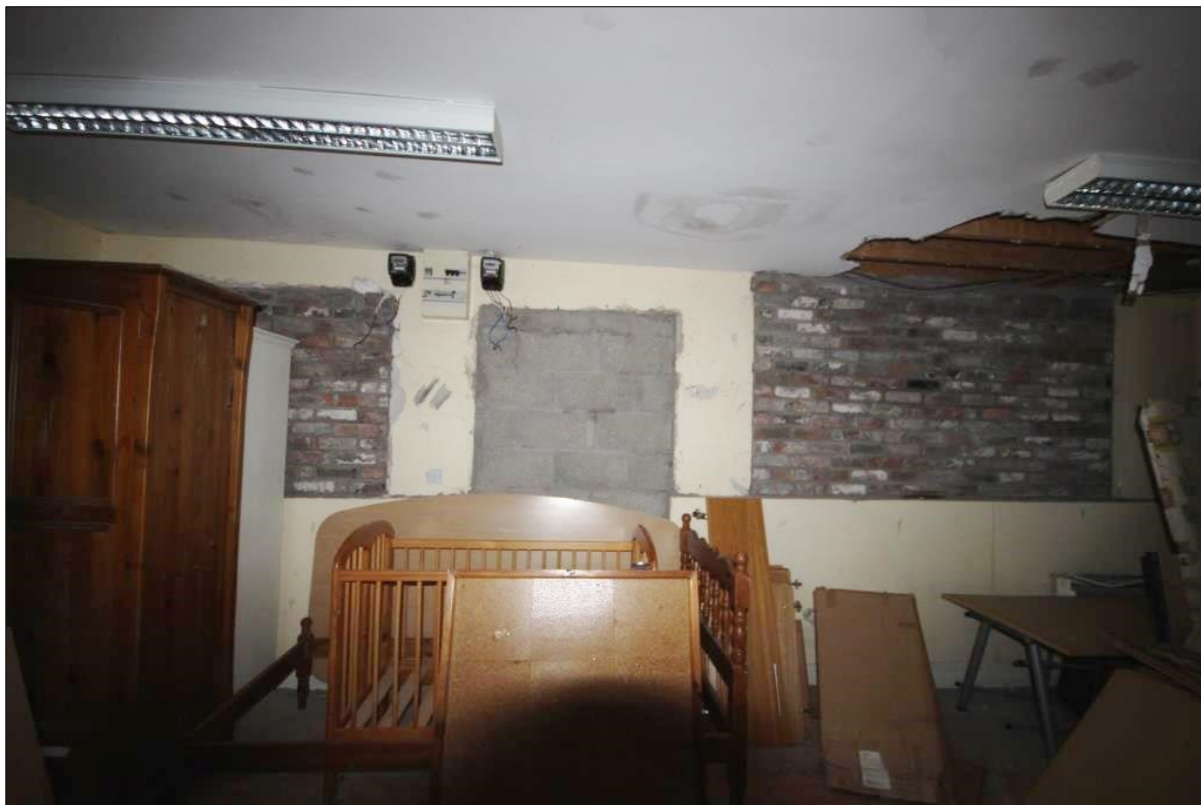
Plate 17: Interior of western wall of Building B with blocked-up openings
