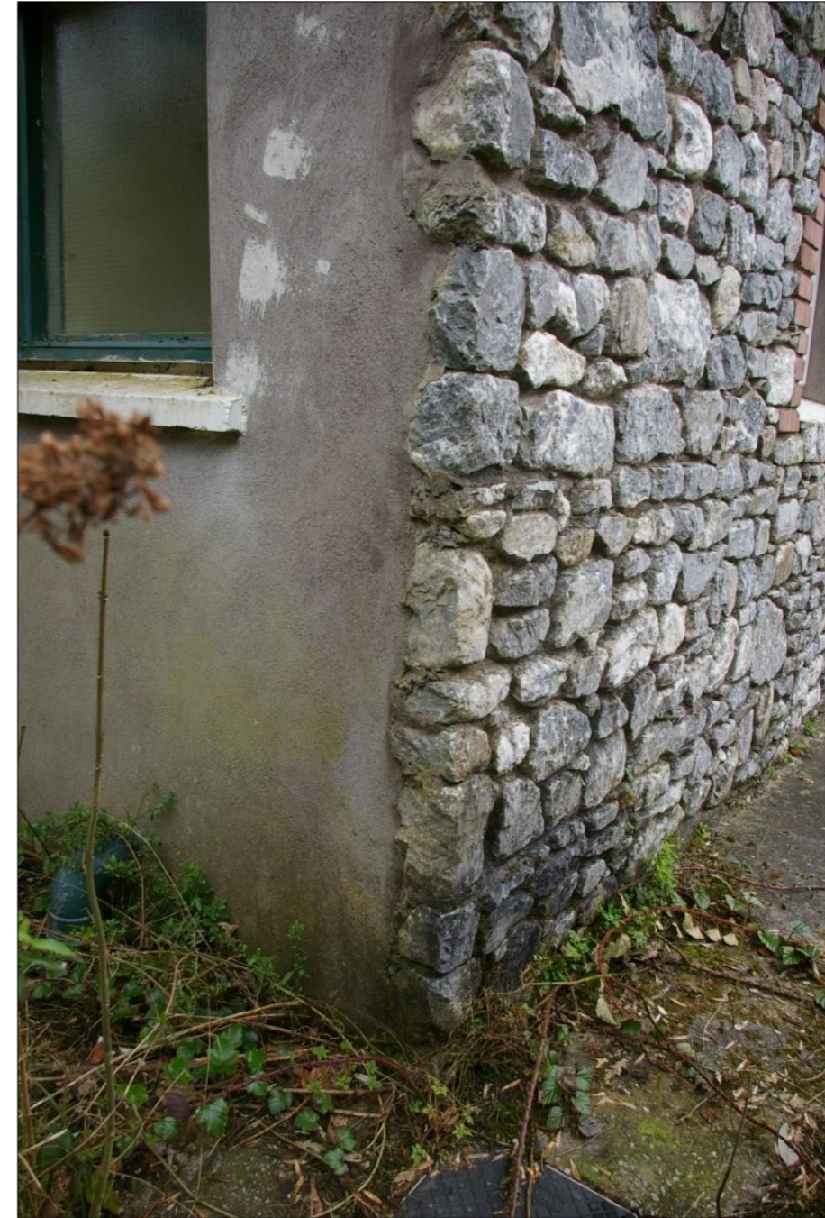
Plate 34: Detail of modern stonework and render on corner of southern elevation of Building G
