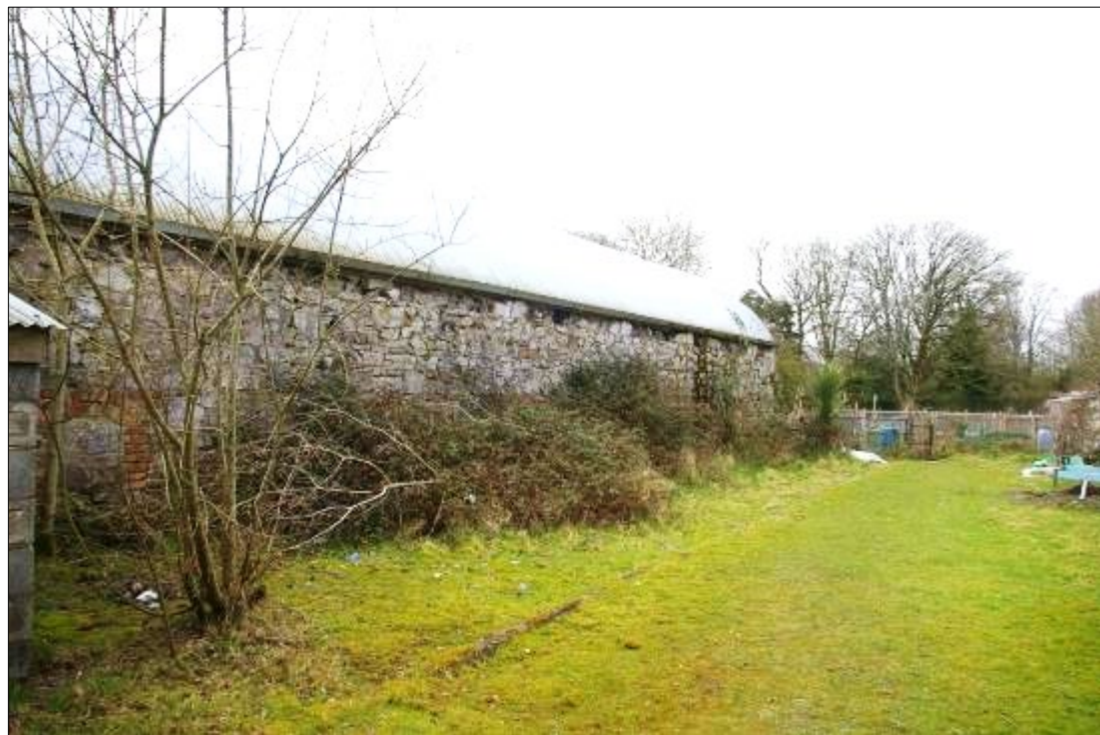
Plate 10.14: Northern elevation of Building C
