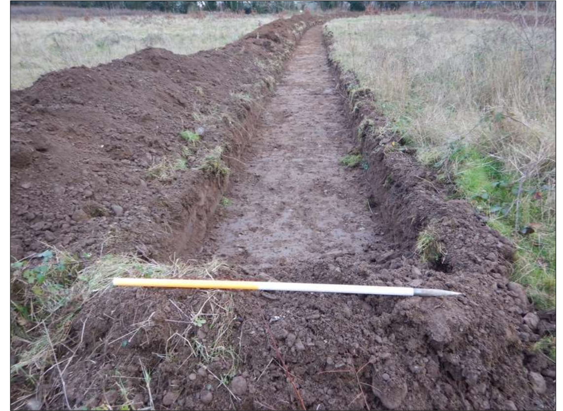
Plate 15 Trench 5, post-ex, looking northeast
