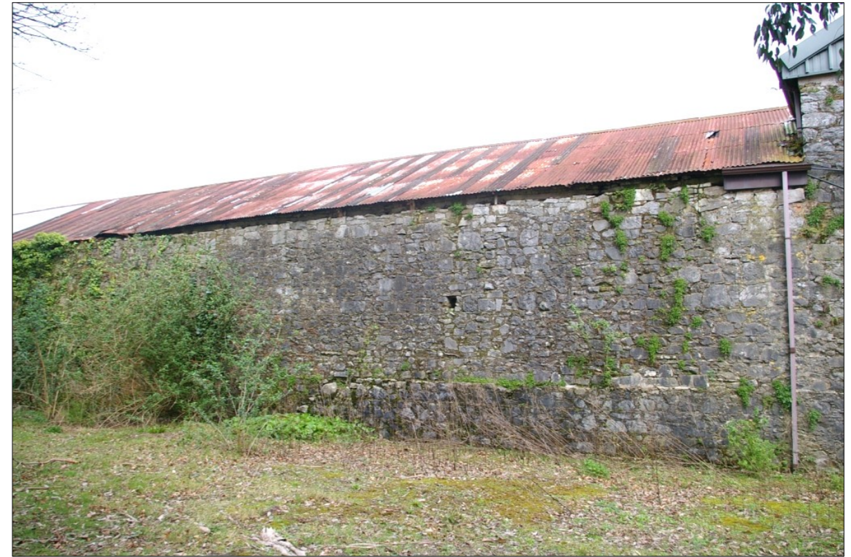
Plate 37: Western elevation of Building H
