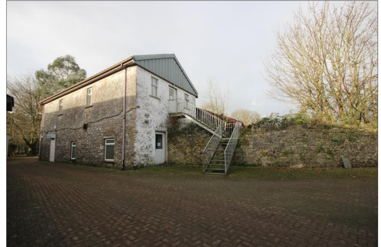
Plate 3: South-eastern and north-eastern elevation of Building A
