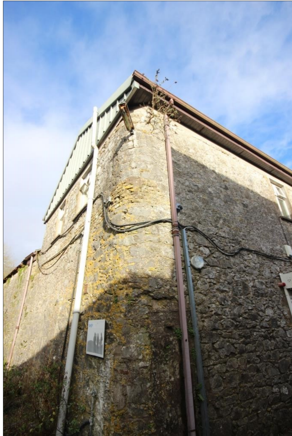
Plate 5: South-eastern corner of Building A
