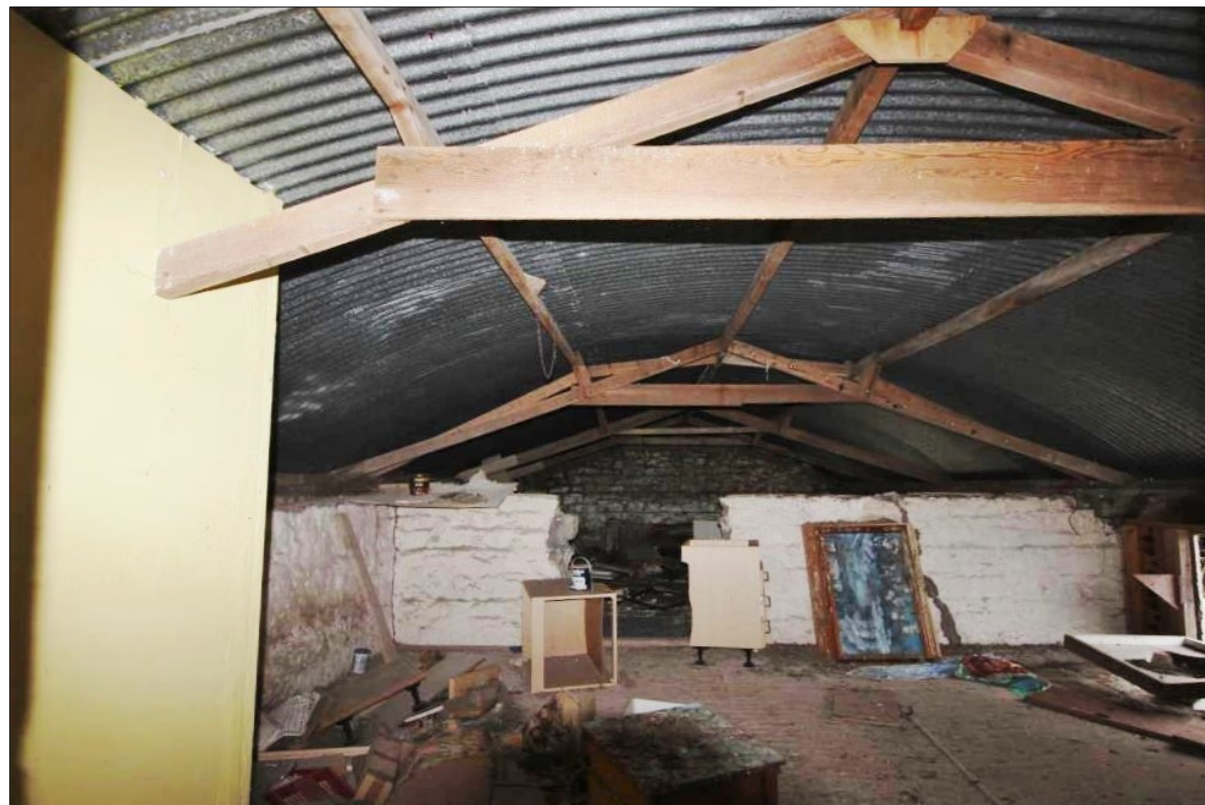
Plate 21: First floor room B-BF Building B
