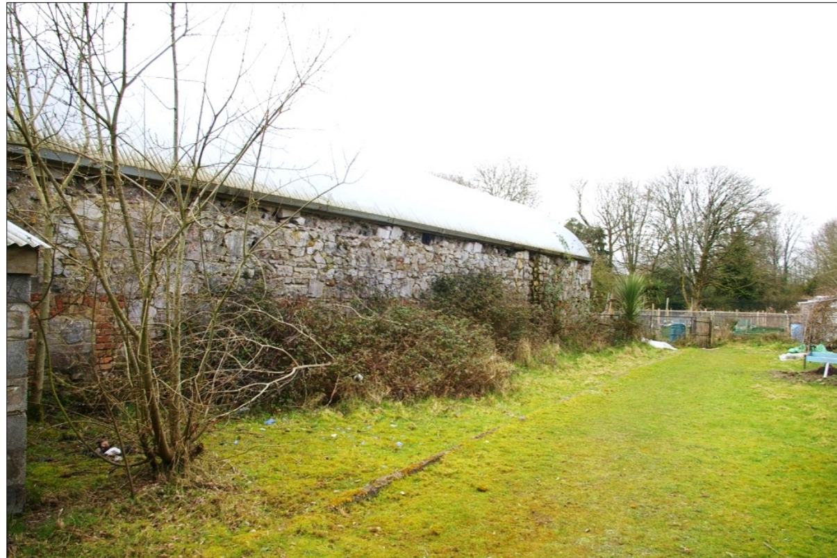
Plate 24: Northern elevation of Building C
