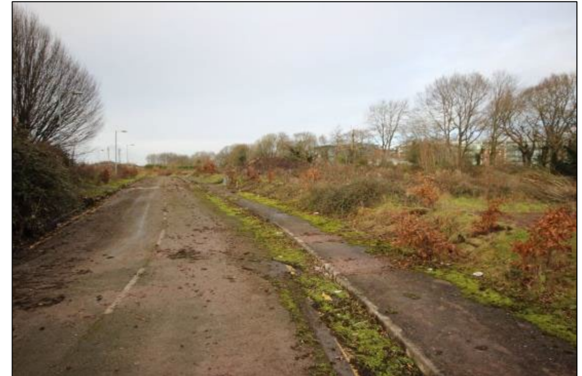
Plate 10.8: Existing road on west side of The Meadows subject lands
