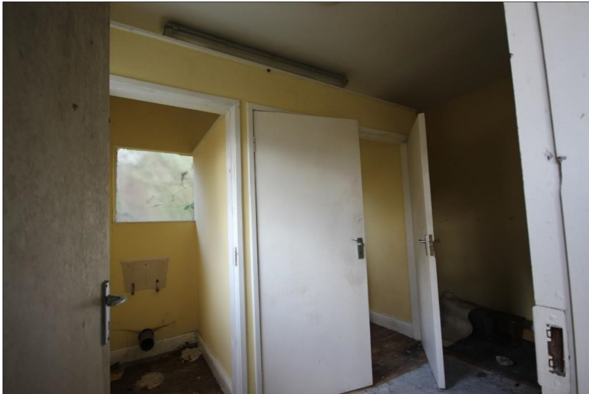
Plate 35: Interior of Building G with modern finishes
