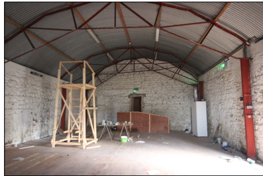
Interior looking south-west
