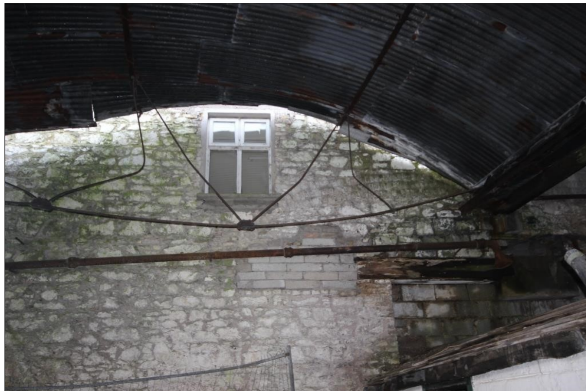
Plate 9: Blocked-up openings in north-western elevation of Building A
