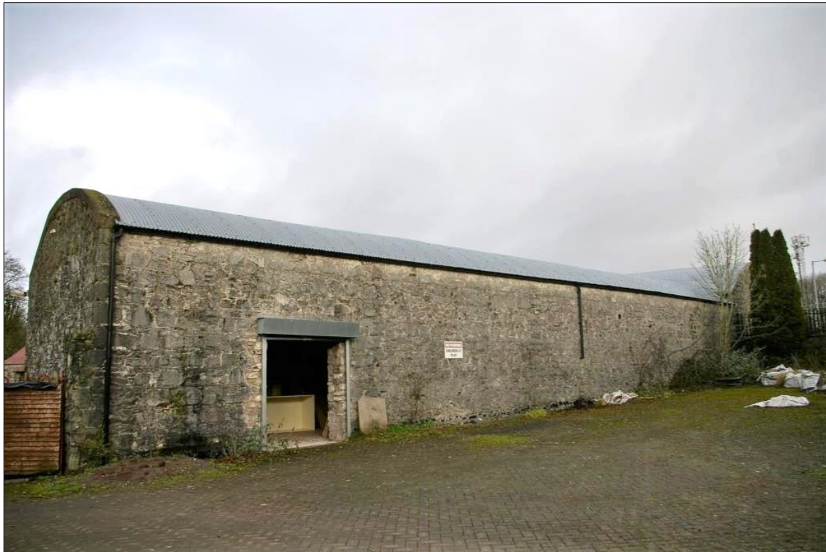
Plate 12: Eastern elevation of Building B
