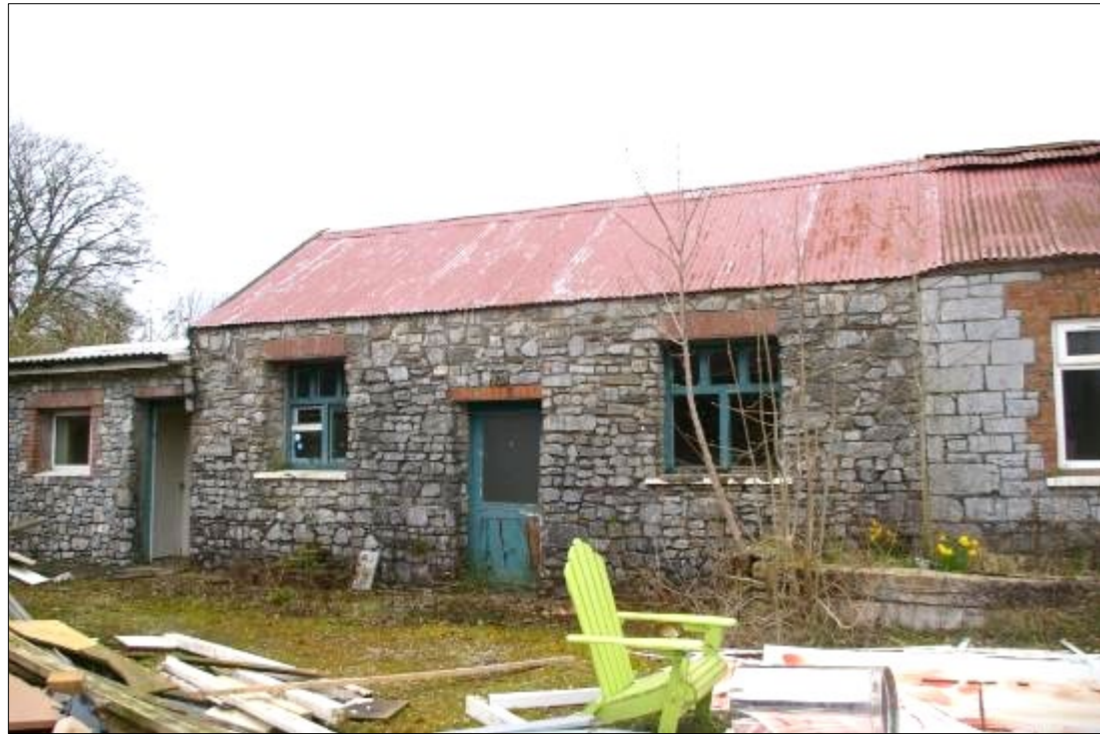
Plate 10.17: Southern elevation of Building F
