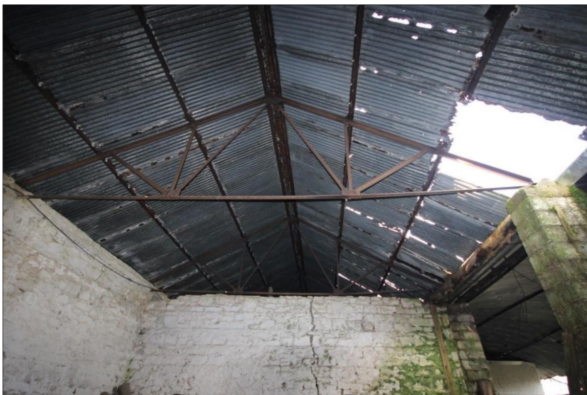
Plate 44: Steel truss roof in eastern section of Building
