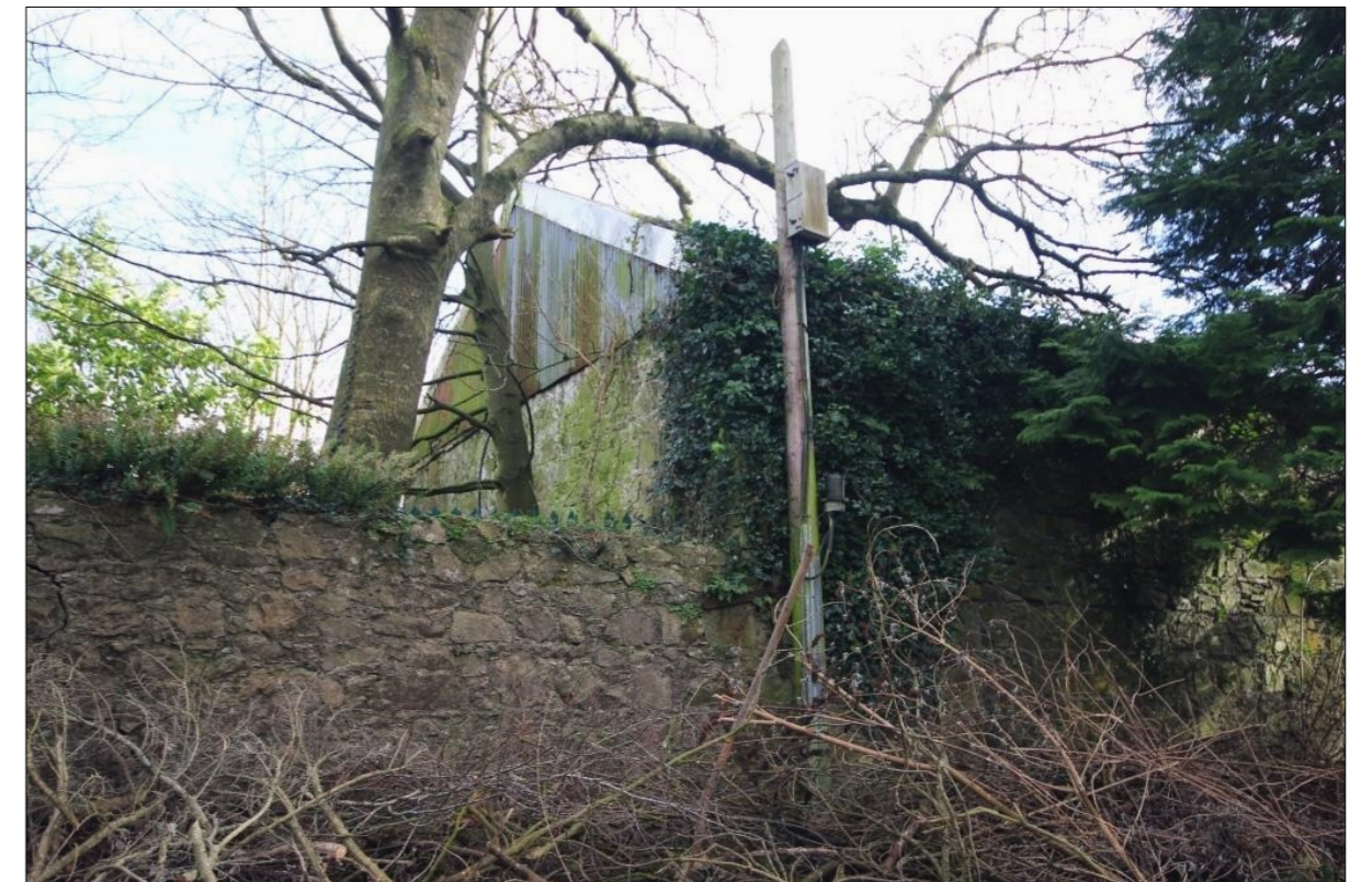
Plate 38: Northern elevation of Building E and boundary wall
