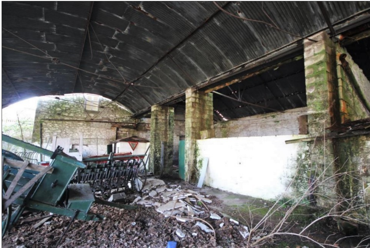
Plate 39: Interior of eastern portion of Building H looking to Building A
