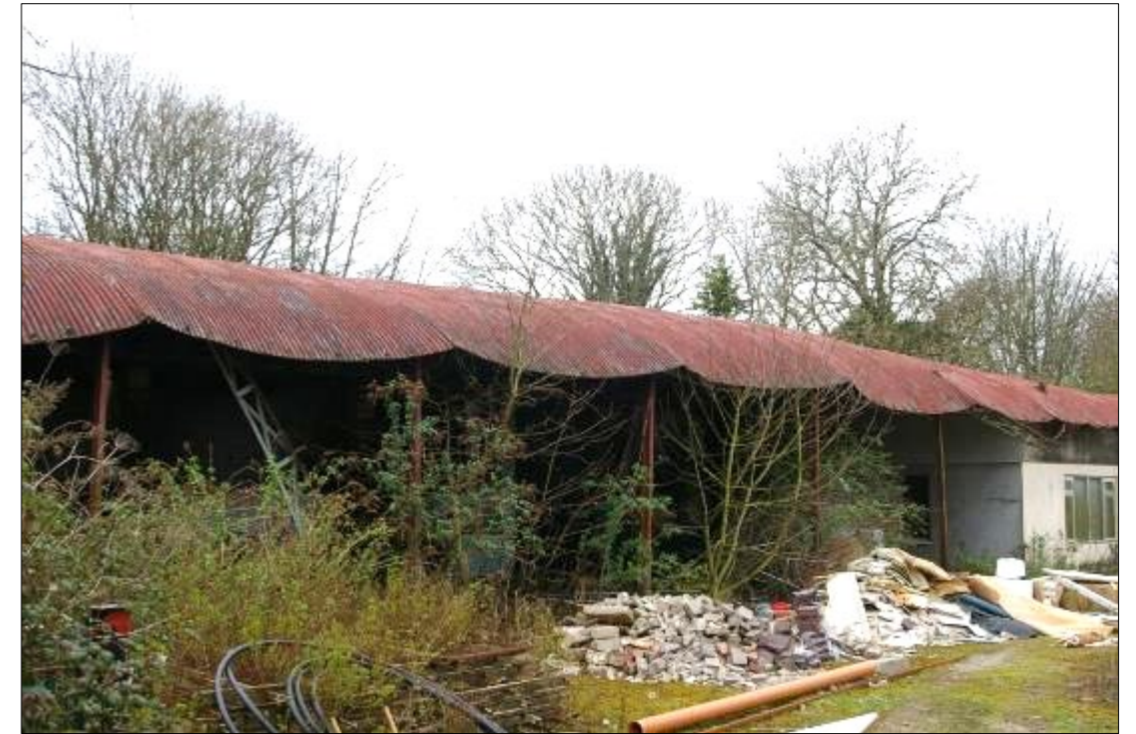
Plate 10.19: Eastern elevation of Building H
