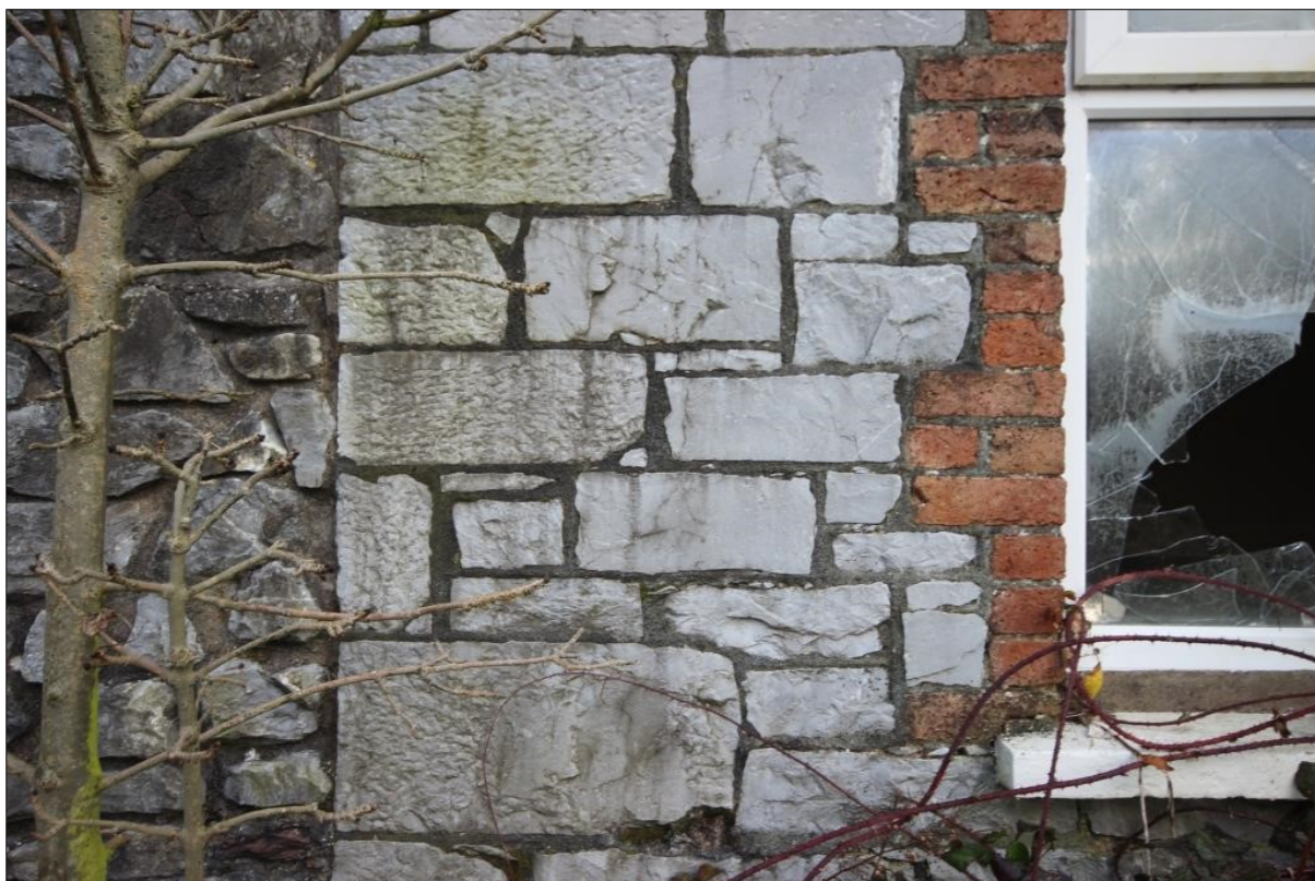
Plate 29: Cut stone detail to wall on southern elevation of Building E
