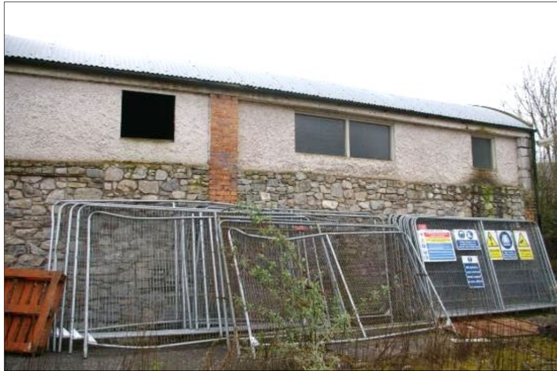
Plate 10.13: Western elevation of Building B. Note upper section rebuilt
