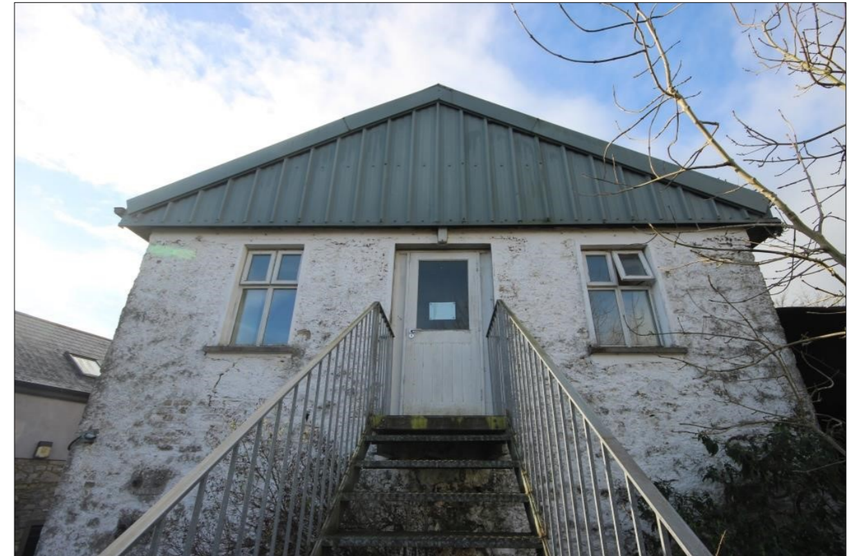
Plate 6: Modern steps to first floor on northeast elevation of Building A
