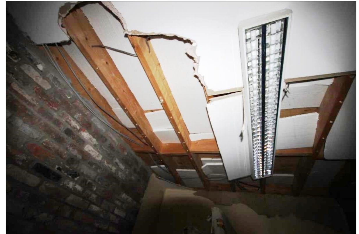
Plate 18: Modern floor joists in Building B
