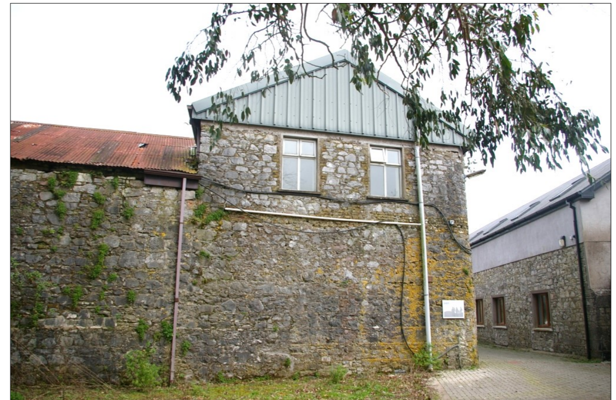
Plate 4: South-western elevation of Building A
