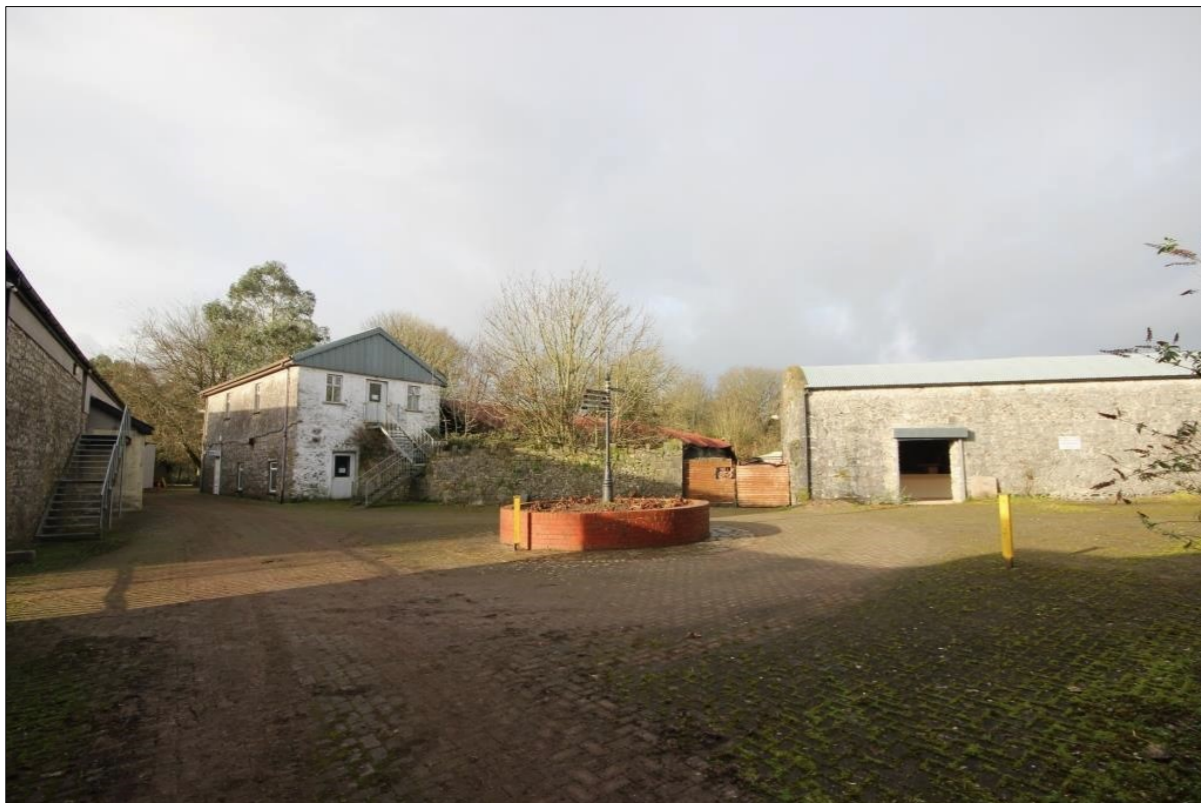
Plate 2: General view to northern range with Building A on left and Building B on right
