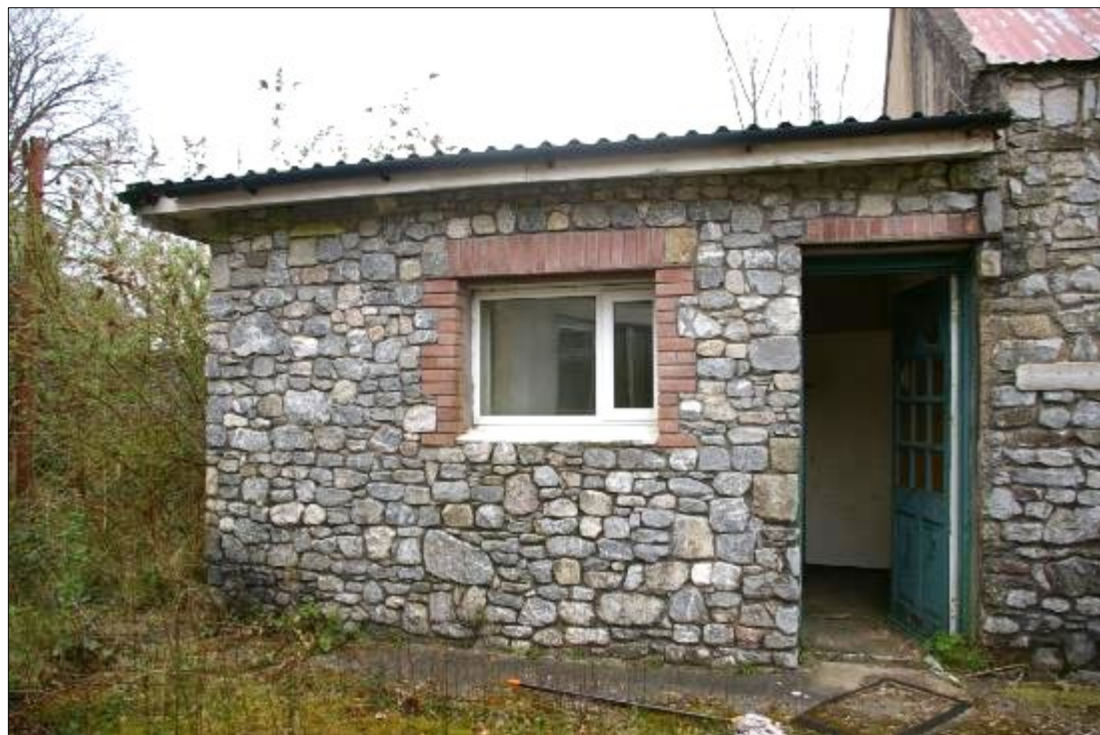
Plate 10.18: Southern elevation of Building G
