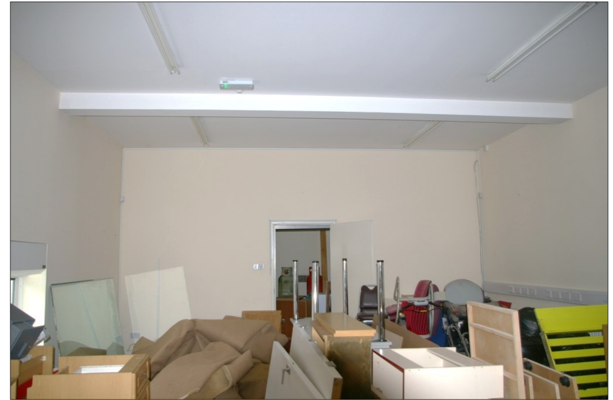
Plate 10: Ground floor room A-GF02 Building A
