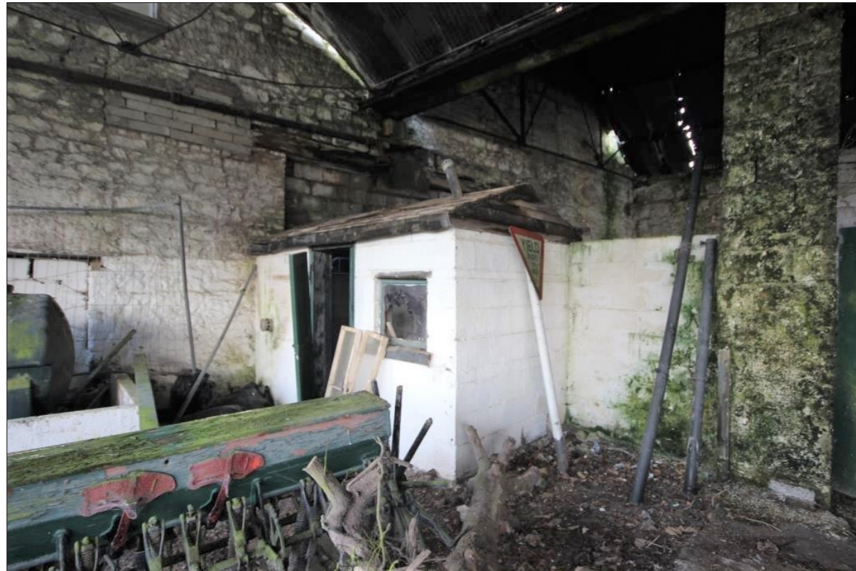
Plate 8: Modern boiler house and north-western elevation of Building A
