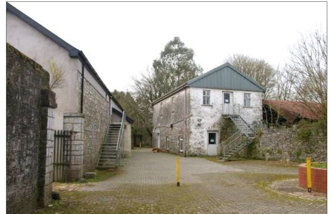
Plate 10.12: South-eastern and north-eastern elevation of Building A within The Farm subject lands
