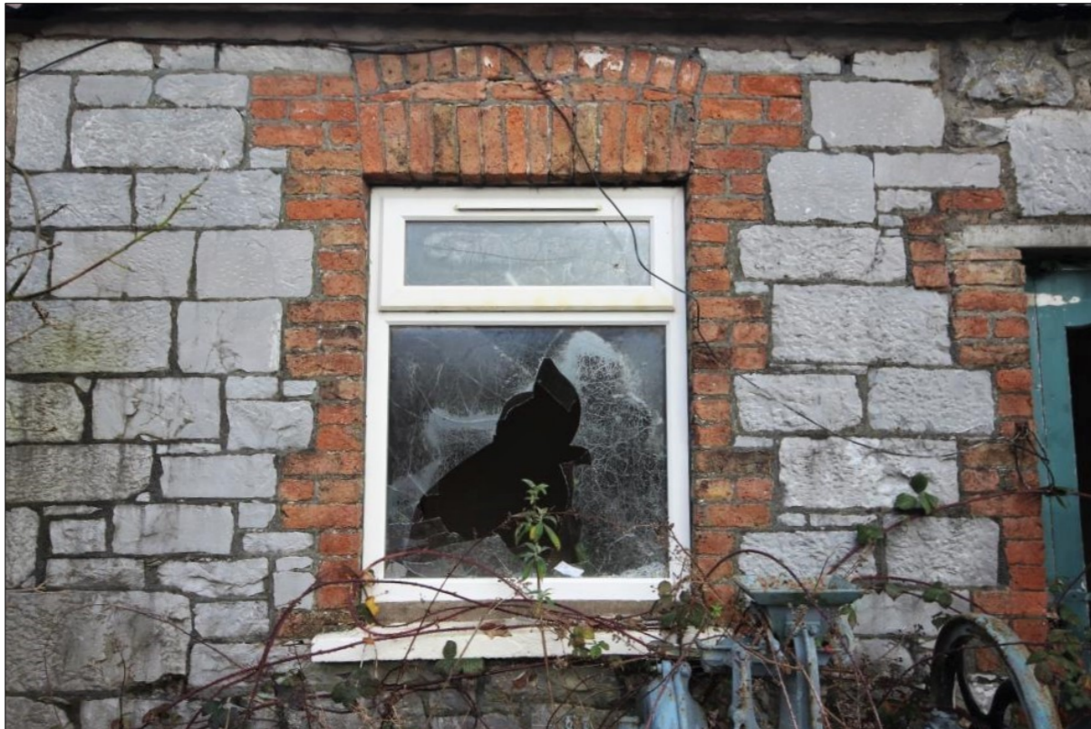
Plate 28: Window detail on southern elevation of Building E with replacement uPVC frame
