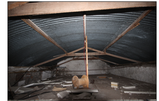
First floor attic space B-FF05
