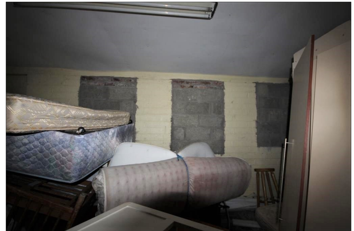
Plate 19: Interior of western wall of Building B with blocked-up openings
