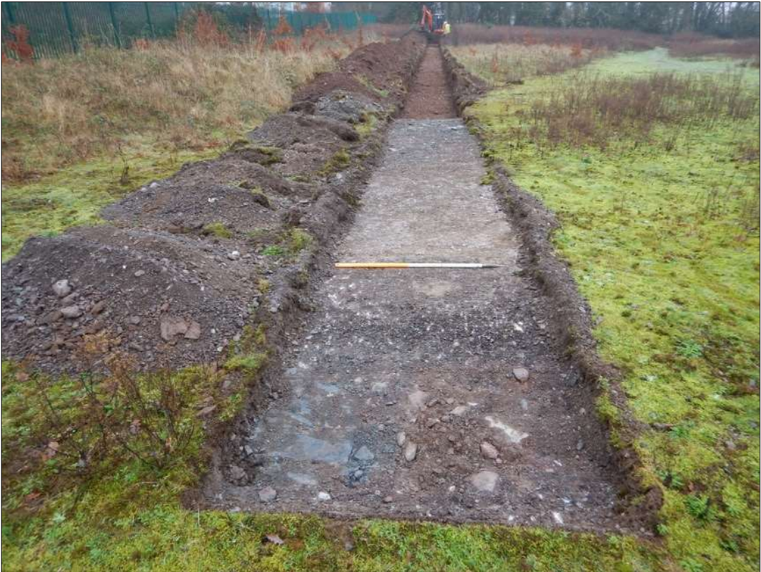
Plate 2 Trench 1, post-ex, looking northeast
