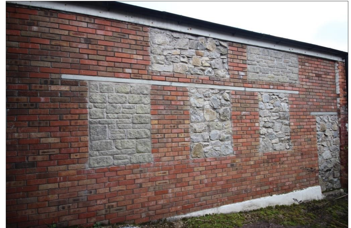
Plate 14: Northern end of western elevation of Building B rebuilt with modern brick and stone finishes
