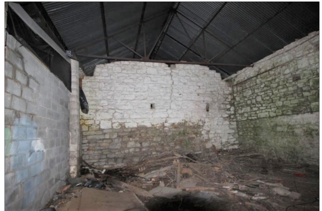
Plate 42: Interior of western section of Building H
