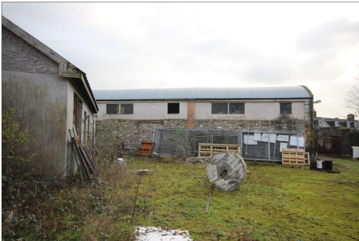
Plate 13: Western elevation of Building B. Note upper section rebuilt
