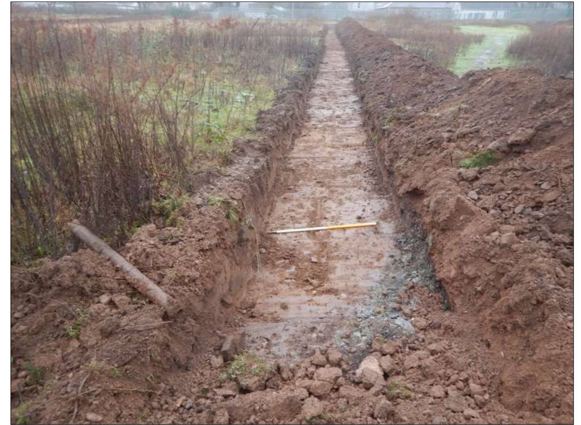
Plate 7 Trench 2, post-ex, looking southwest
