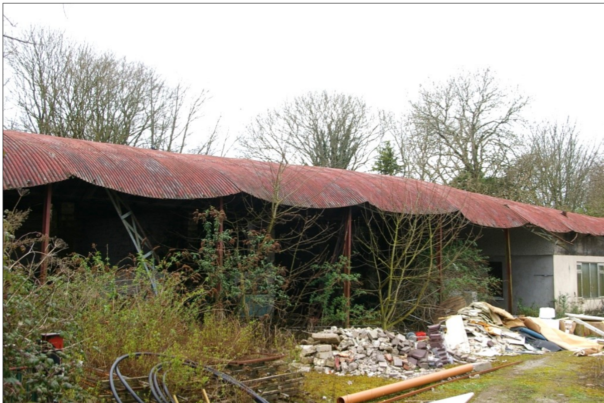
Plate 36: Eastern elevation of Building H
