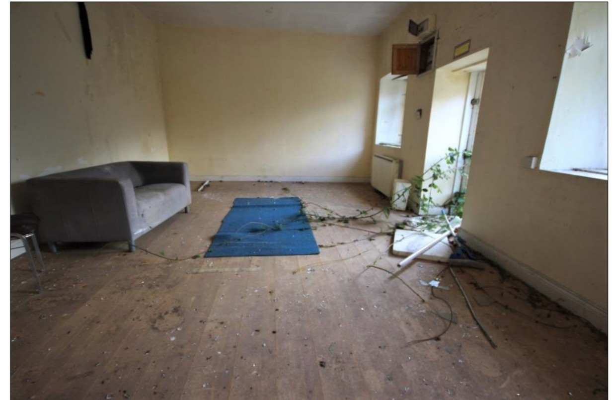
Plate 30: Interior view of Building E with modern floor, ceiling and wall finishes
