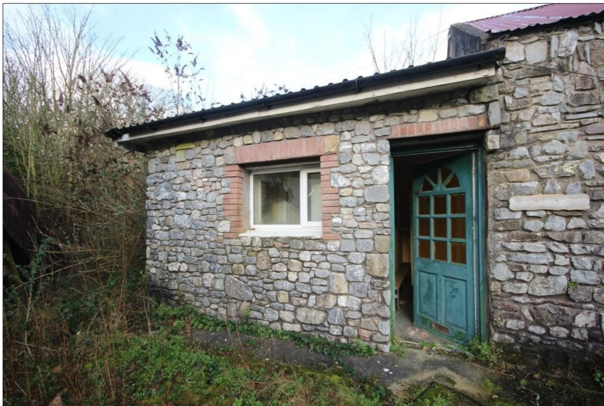
Plate 33: Southern elevation of Building G
