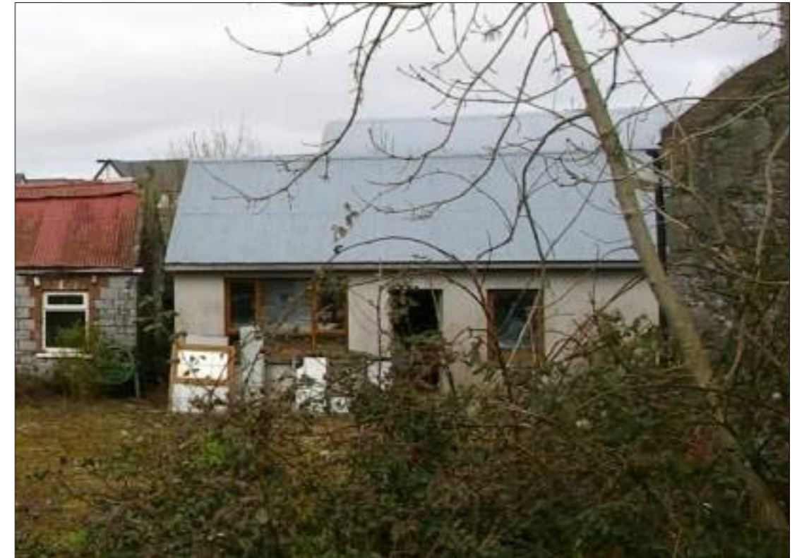
Plate 10.15: Southern elevation of modern structure Building D
