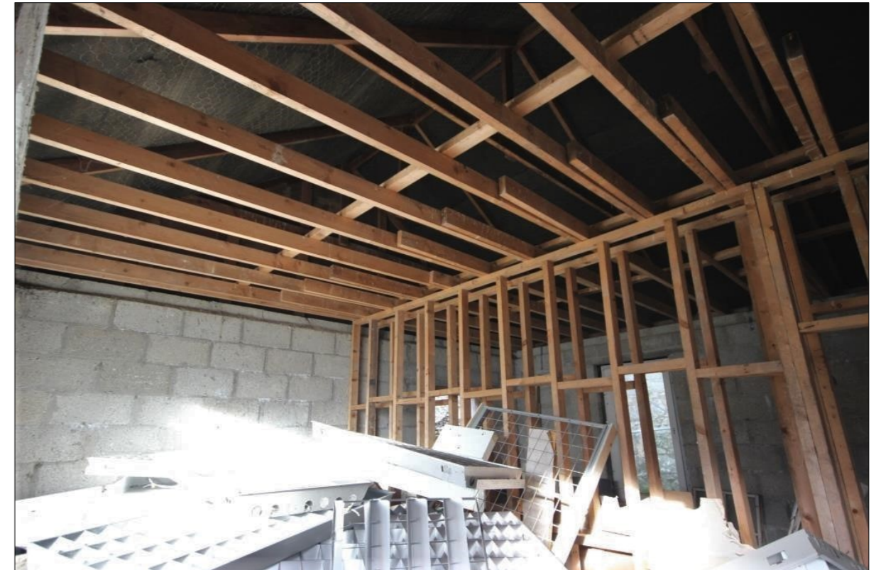
Plate 26: Interior of Building D with modern blockwork and joinery
